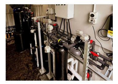
We designed and installed an innovative containerised water treatment plant that is compact and produces excellent water quality. Equipped with advanced technologies such as multimedia filtration, carbon filters, softeners, ultra-filtration (UF), UV treatment, and chlorine dosing, this combination ensures the highest quality water treatment, effectively removing fine materials and contaminants, especially during severe weather events.
