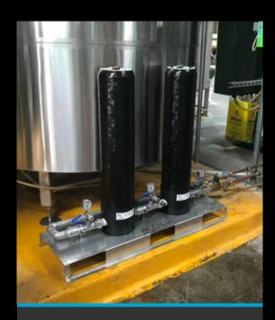
"The cartridge from this system has a volume that is 8 times greater than standard 20" Jumbo filters."
