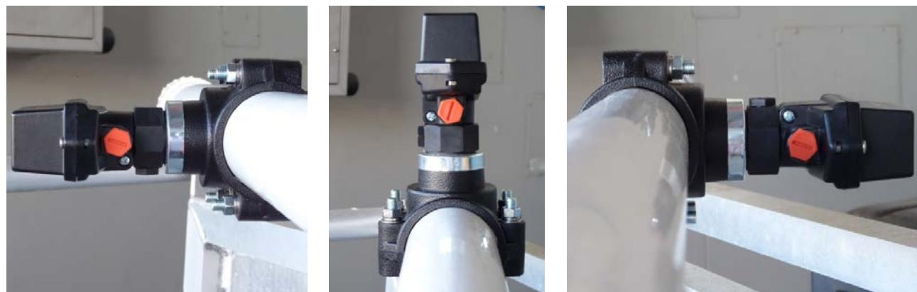
The flow switch should not be mounted on the underside of horizontal pipes.
